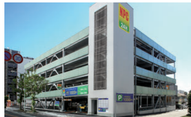
Parking lots that efficiently utilize land by creating multi-level floors
