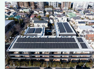
Solar panels installed across the entire rooftop of the property
